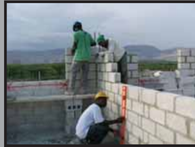
More wall construction
