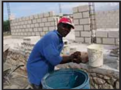
Building the walls
