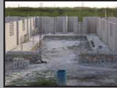
Inside view of walls
